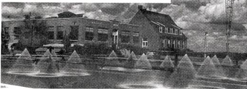
WLW transmitter plant at Mason, O. The spray pond in the foreground pumps a million gallons daily. The 500,000-watt transmitter building is at left, with operator's dormitory in center, 830-foot radiator, in rear.
